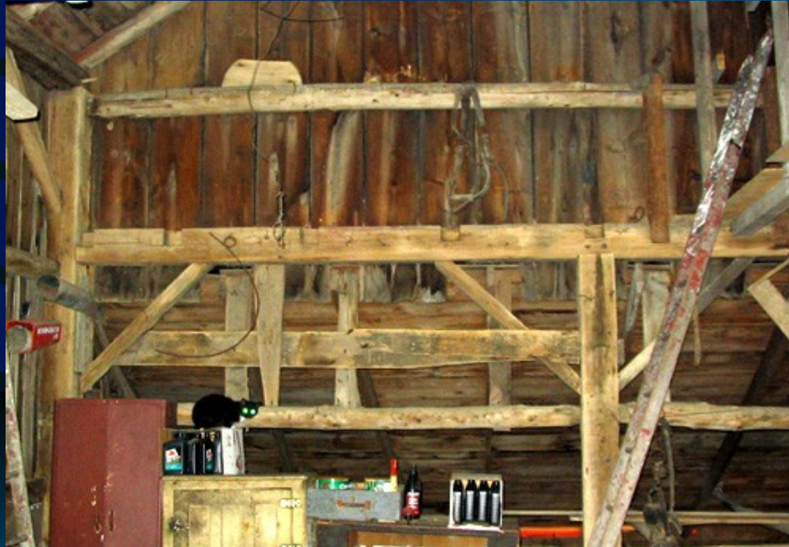
Twin Pines Farm barn interior, Concord Center Drive
