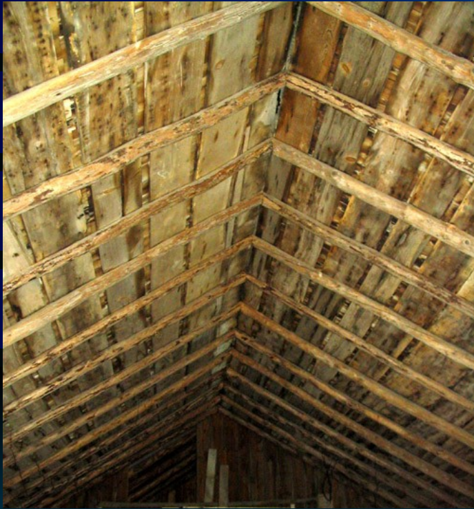
Twin Pines Farm tamarack rafters Concord Center Drive
