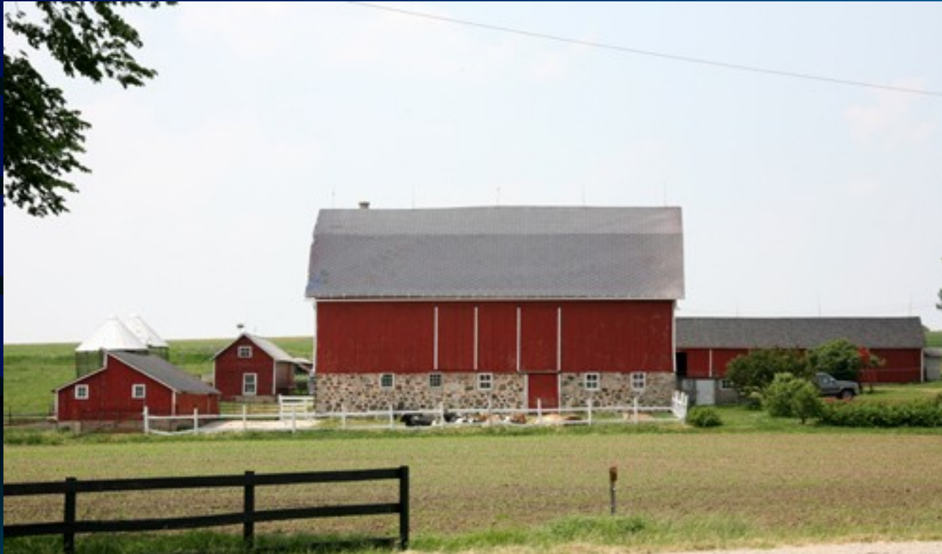
Pitterly Farm, Barns and Out Buildings, Hwy. E
